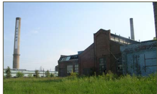
Site Building – August 2008
